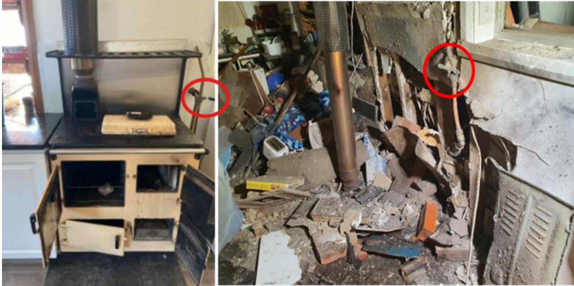
Before and after: A slow-combustion stove with wetback water jacket (note the isolation valve)
