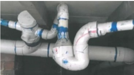
Example of non-compliant plumbing work
