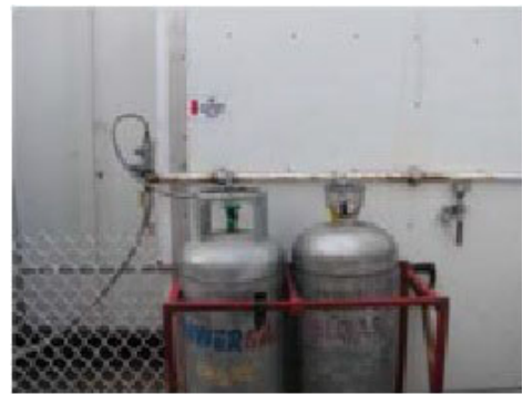
Secured and clear of combustibles
