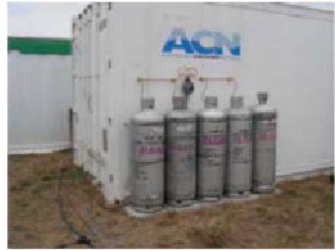
Secured and on a stable base
