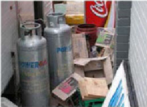
Not clear from combustibles or secure
