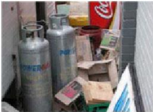
Not clear from combustibles or secure
