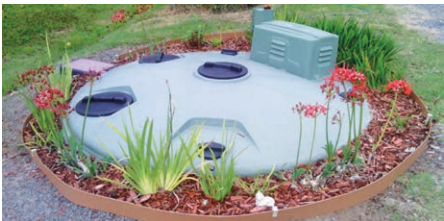
Example of an On-site domestic wastewater treatment system
